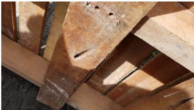
Dunnage within the container baring holes
